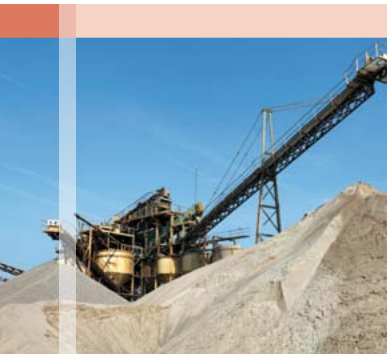
Gravel works with conveyor system at the Straberger Baggersee Lake, Dormagen
