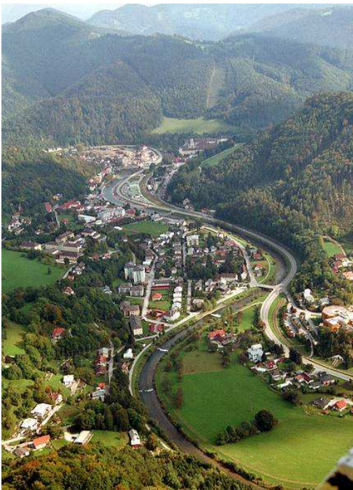
Upper part of the basin at Lilienfeld
