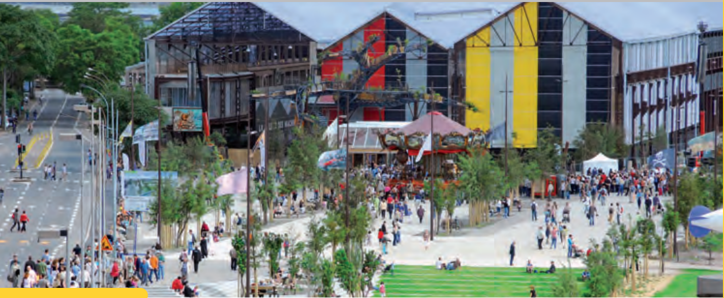
Construction site on Nantes Island - Photo Credits Vincent Jacques
