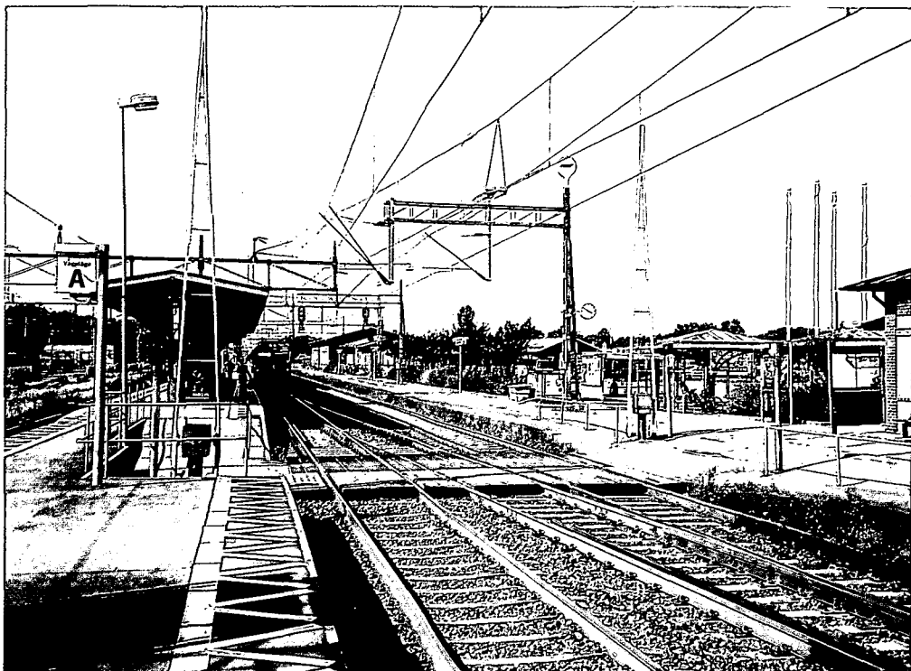
Photo 5.15 Angleholm Station (Sweden) - level crossing
