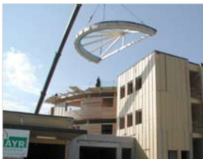
The prefabricated building's wooden structure and its cladding were assembled in just nine days.
