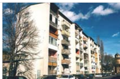
The Daungasse estate before award-winning retrofitting and renovation.
