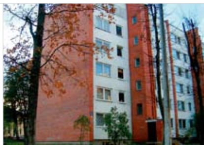
The 139 multi-storey apartment buildings were energy-rated.
