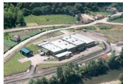
The biogas produced by the pilot plant has a methane content of around 80%.
