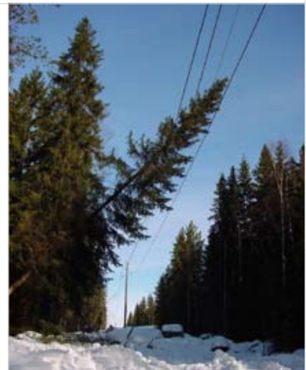
The developed fault indication system detected fallen trees on the power line in different environmental conditions and seasons.
