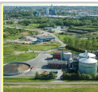
Figure 10: Since 1997, the biogas production unit of Svensk Biogas AB in Linköping has been capable of processing 100 000 tonnes of waste (mainly from slaughterhouses) to obtain 4.7 million m 3 of biogas (97% CH 4 ). The gas is compressed to 250 bar and is used in urban buses (the entire fleet using biogas), passenger cars (12 stations) and the first train running on biogas in the world. 16
