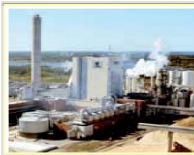
Figure 9: Built in 2004 the Wisa Power plant can use black liquor as a source of energy by burning it to produce both heat (600 MW used for the production of paper pulp) and electricity (140 MW). This is one of the largest facilities of its kind in the world. 10
