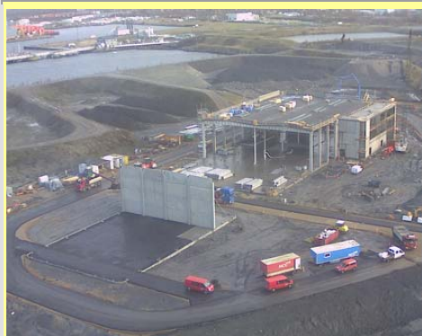
Figure 17: Construction on the Kalunborg site in 2008 (Inbicon project). After an initial mechanical treatment, the wet straw is heated to about 200 ° C for 5 to 15 minutes to destroy the structure made of lignin and make the cellulose accessible to the enzymes then added. After this pre-treatment, there remains the classical stage of fermentation. The installation should be commissioned in late 2009 and produce 4 500 tonnes of ethanol, 8 250 tonnes of solid fuel and 11 000 tonnes of
